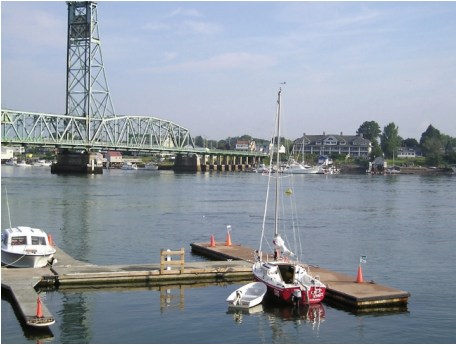
Strong currents sweep beneath Memorial Bridge - Prescott Park Dock, Portsmouth, NH
