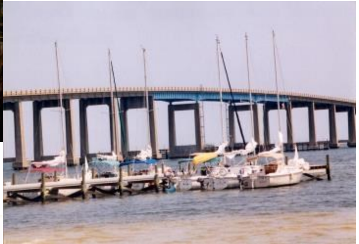
The free T-dock at Navarre has long been a favorite place to "take a break" between Spectre Island and Pensacola Beach, both westbound and eastbound (though thanks to an inconsiderate power boater, who damaged several boats here with his wake during the 2014 NGCC, future cruisers may have second thoughts about stopping here).
